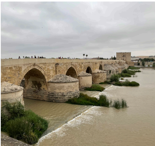
Roman Bridge, Cordoba
